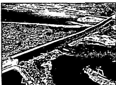
The S.R. 46 project involved design of a new bridge and removal of an existing causeway at Lake Jesup.
